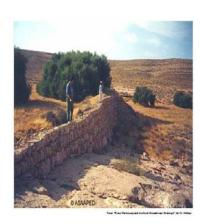
Jessours in the Matmata moutains. A hydraulic unit made of three components: the catchment area, the terrace and the dyke. The jessours are used to bank the runoff from the mountain chain.
